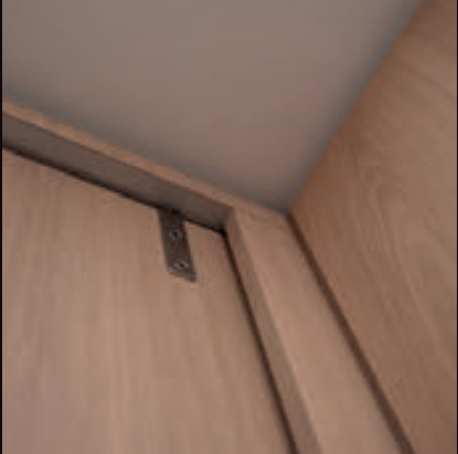
Flow veener stainless steel pivot
