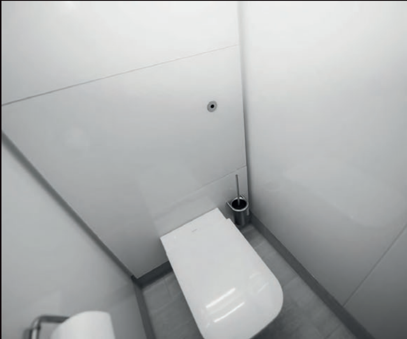
Sentry glass IPS with WC pan highlighting hinged opening
