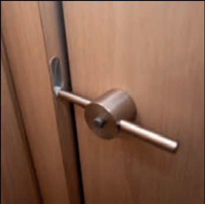
Flow veener lock locates in receiver
