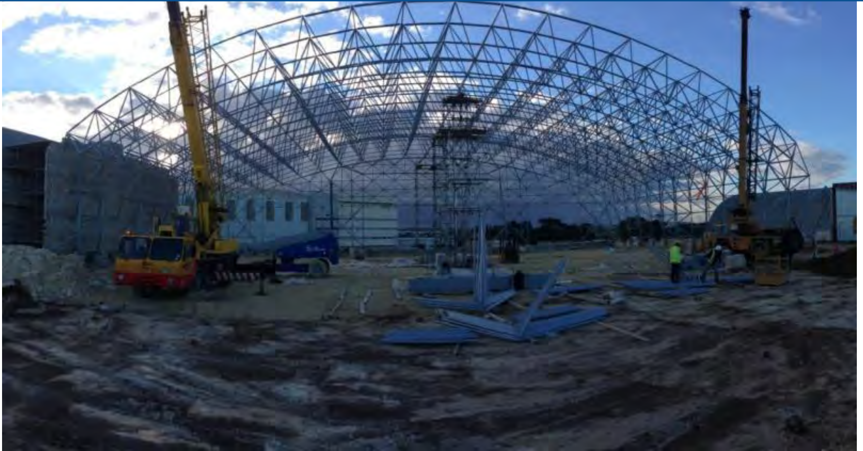
MALTA AIRCRAFT HANGAR - Vault - 2014 - Malta 2.500 m 2 x 3 units Span 60 m
