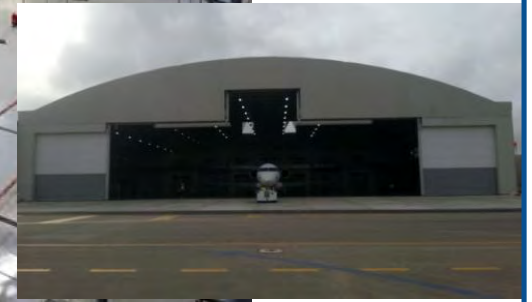
MALTA AIRCRAFT HANGAR - Vault - 2014 - Malta 2.500 m 2 x 3 units Span 60 m
