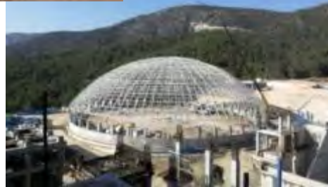
Dinçer Çimento Preblending Unit - 2018 - Bilecik - TURKEY 8.450 m 2 Height 25 m Diameter 88 m
