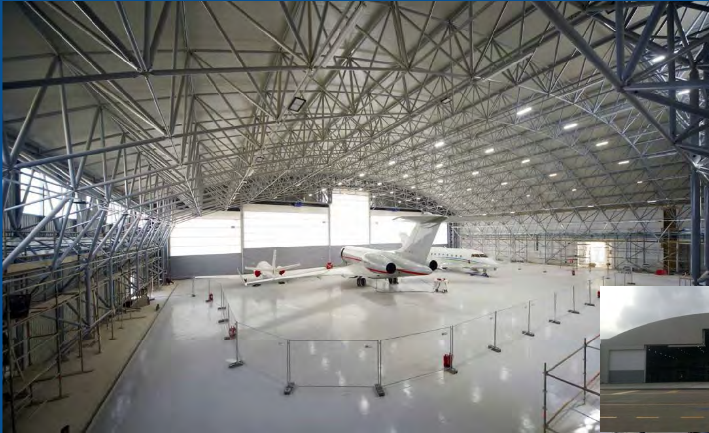
MALTA AIRCRAFT HANGAR - Vault - 2014 - Malta 2.500 m 2 x 3 units Span 60 m
