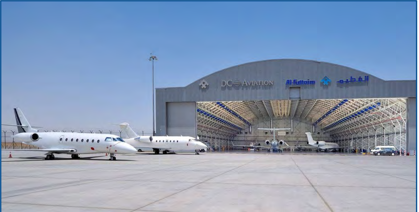
Dubai Aircraft Hangar - Vault - 2012 - Dubai / UAE 6.800 m 2 Span 65 m
