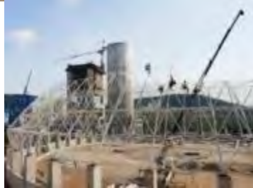
Dinçer Çimento Preblending Unit - 2018 - Bilecik - TURKEY 8.450 m 2 Height 25 m Diameter 88 m
