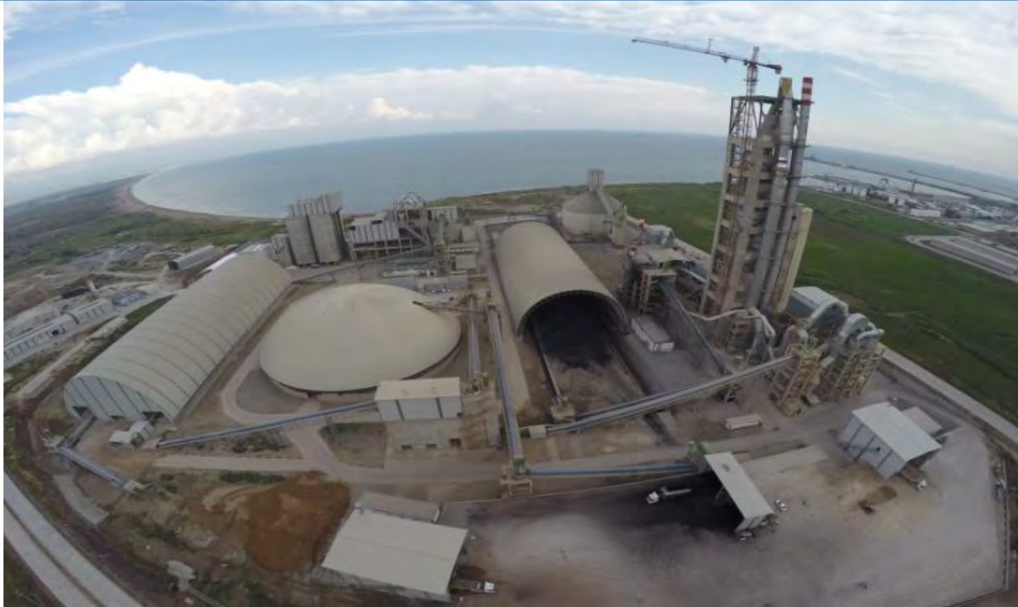
Preblending & Additive Storages - 2013 - İskenderun / TURKEY 45.000 m 2 Spans 52 m & Diameter 98m
