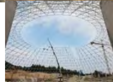
Dinçer Çimento Preblending Unit - 2018 - Bilecik - TURKEY 8.450 m 2 Height 25 m Diameter 88 m
