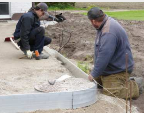
Profile 120 mm with concrete-/earth-anchor and connector
