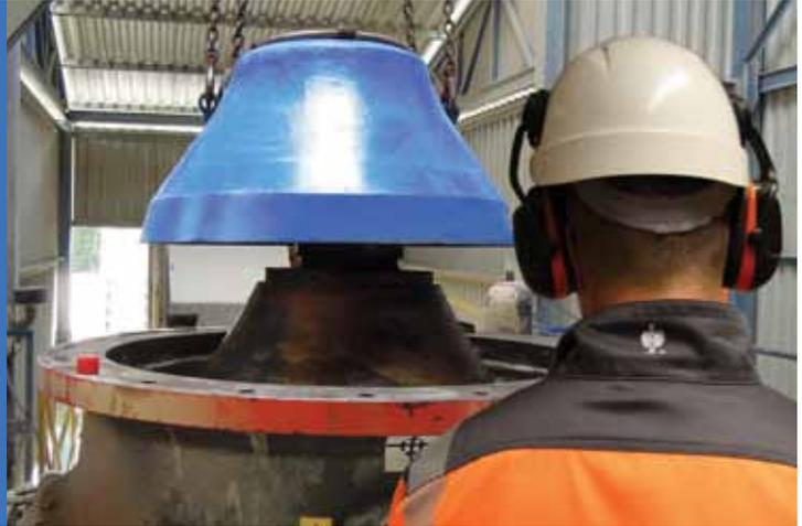
CMS Cepercor™ are a leading supplier to UK quarrying groups for scheduled cone crusher liner changes and servicing, minimising downtime and ensuring cost effective operations.
